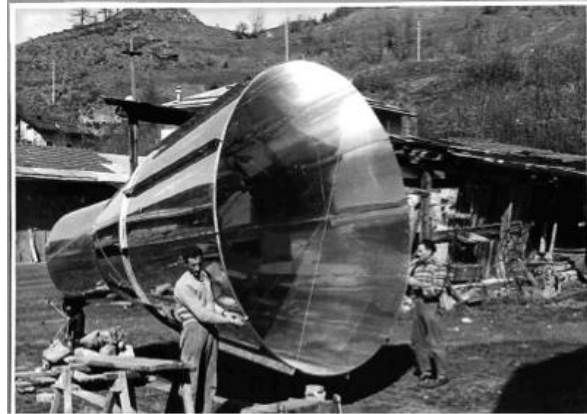
Fig. 5. The initial Francia cone collector. Source: Italian Group for the History of Solar Energy (GSES)
