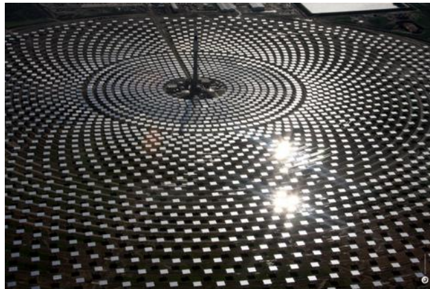
Fig. 10. Spanish 20 MW(e) Gemasolar PT plant with 15 hours of molten salt storage. Source ref [12].
