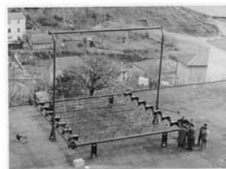
Fig. 2: Frame supporting structure of the first Fresnel Linear Reflector, designed by Giovanni Francia and installed in cooperation with Marcel Perrot in Marseilles in 1963 (Photo courtesy of the Francia heirs).
