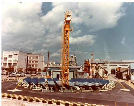
Fig. 13 Solar tower plant built at Georgia Tech, in Atlanta (U.S.), with the collaboration of Ansaldo and Giovanni Francia
