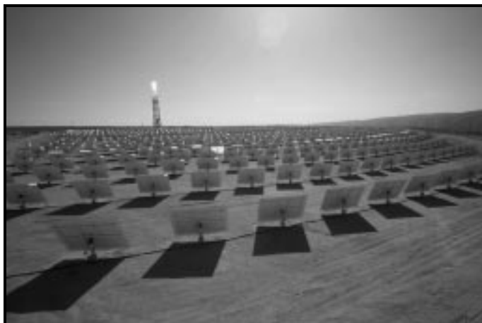
Fig. 17. 6 MWth Luz Power Tower (LPT), in the Negev desert (Israel), put in service by BrightSource Energy in 2008 (Source: Photo courtesy of BrightSource Energy).
