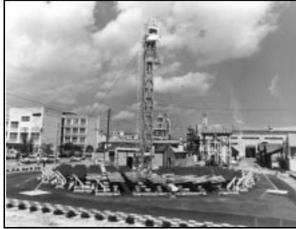
Fig. 12. Solar tower plant built at Georgia Tech, in Atlanta (US), with the collaboration of Ansaldo and Giovanni Francia (Source: Photo courtesy of the G. Parodi archives, 1979).
