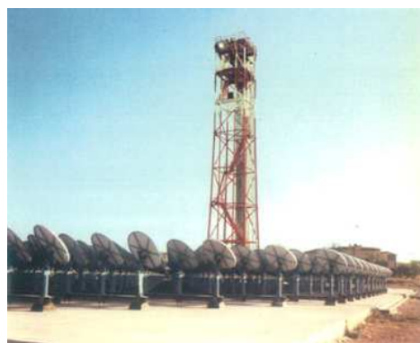
Fig. 14 The Eurelios plant, view of the heliostat field and the boiler tower Source: Photo courtesy of the G. Parodi archives, 1982
