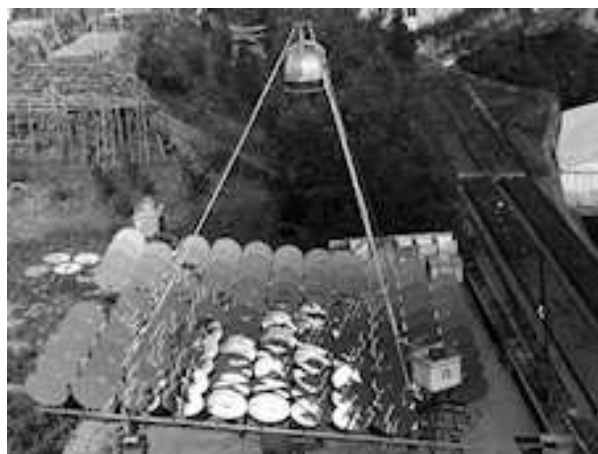
Fig. 12 - World's first solar tower plant, with field of point-focus Fresnel mirrors, built and tested at Sant'Ilario, near Genoa (Italy), in 1965 Source: Photo from the Giovanni Francia archive, donated by his heirs to the Museum of Industry and Labor, Brescia
