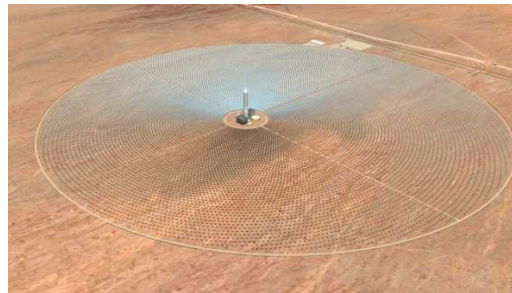
Fig. 21 – Left - Scheme of a new type of solar-power plant that will use molten salt to store the sun's heat so it can be converted to electrical power even when the sun isn't shining creating utility-scale storage technology. Right – A model rendering of Solar Reserve plant at Crescent Dunes, near Tonopah, Nevada – Source: Images courtesy of Solar Reserve
