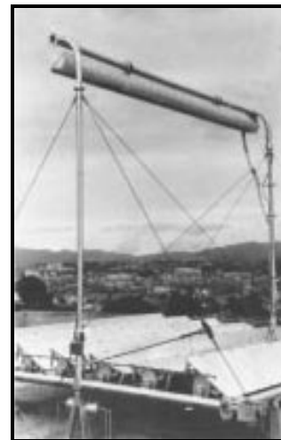
Fig. 10. World's first linear Fresnel concentration-type solar plant, built and tested at Marseilles (France) in 1963 (Source: Photo from the Giovanni Francia archive, donated by his heirs to the Museum of Industry and Labor, Brescia).
