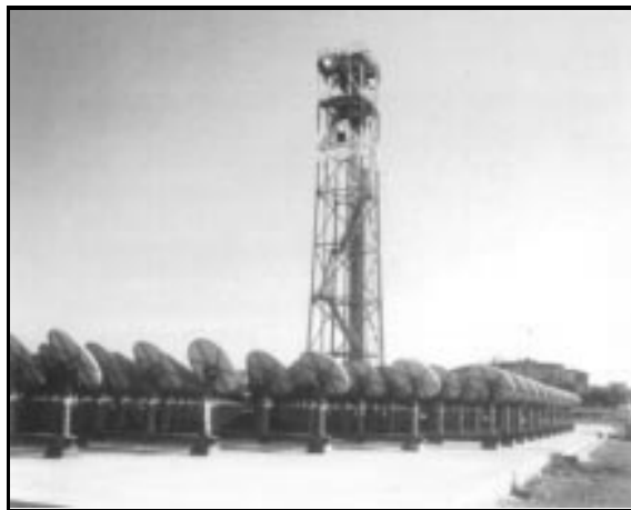
Fig. 14. "La Capanna" experimental solar station at ENEA's Casaccia Research Center (Source: Photo courtesy of ENEA, 1983).
