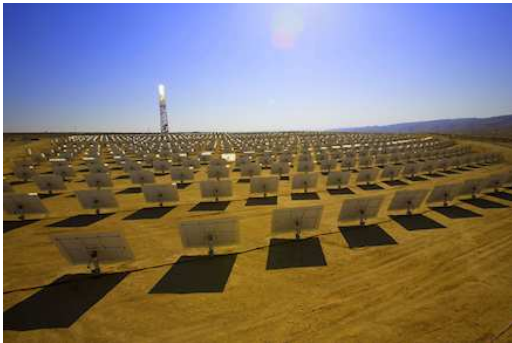
Fig. 18 – 6 MWth Luz Power Tower (LPT), in the Negev desert (Israel), put in service by BrightSource Energy in 2008. - Source: Photo courtesy of BrightSource Energy
