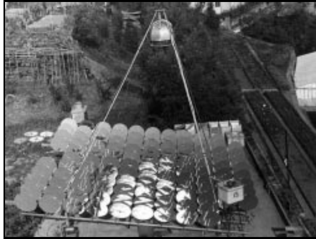
Fig. 11. World's first solar tower plant, with field of point-focus Fresnel mirrors, built and tested at Sant'Ilario, near Genoa (Italy), in 1965 (Source: Photo from the Giovanni Francia archive, donated by his heirs to the Museum of Industry and Labor, Brescia).
