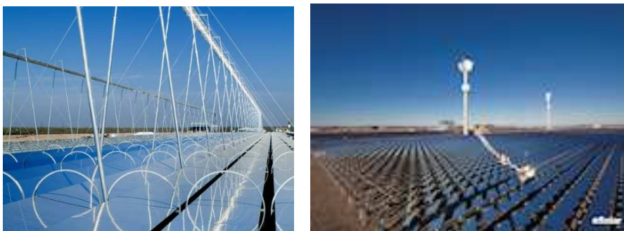
Fig. 16 Areva Solar (formerly Ausra) 5 MWe Kimberlina solar plant, put in service in 2008
