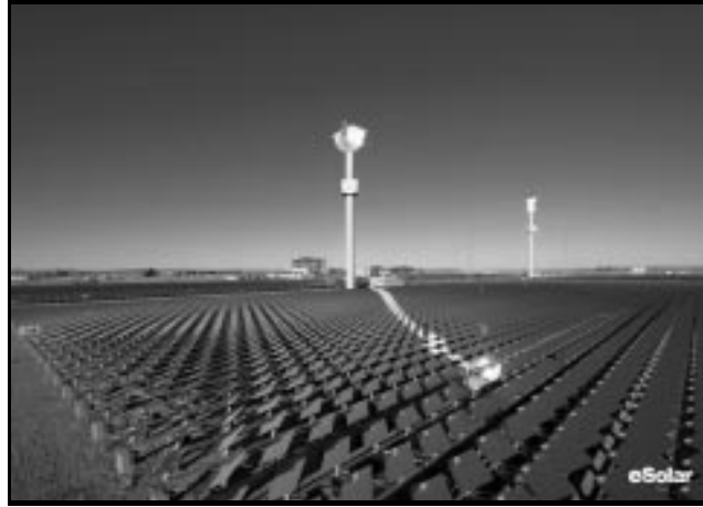
Fig. 16. e-Solar 5 MWe Sierra Sun-Tower, put in service in 2009 (Source: Photo courtesy of eSolar).
