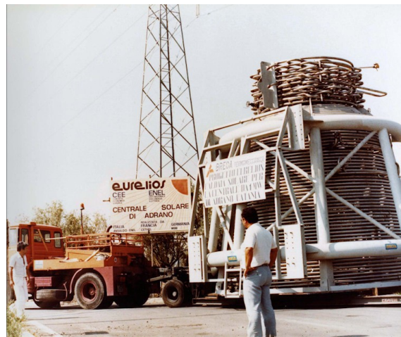
Fig. 12: Eurelios' solar boiler before its installation on the top of the tower, photo 1980, MUsil, Brescia, Italy.
